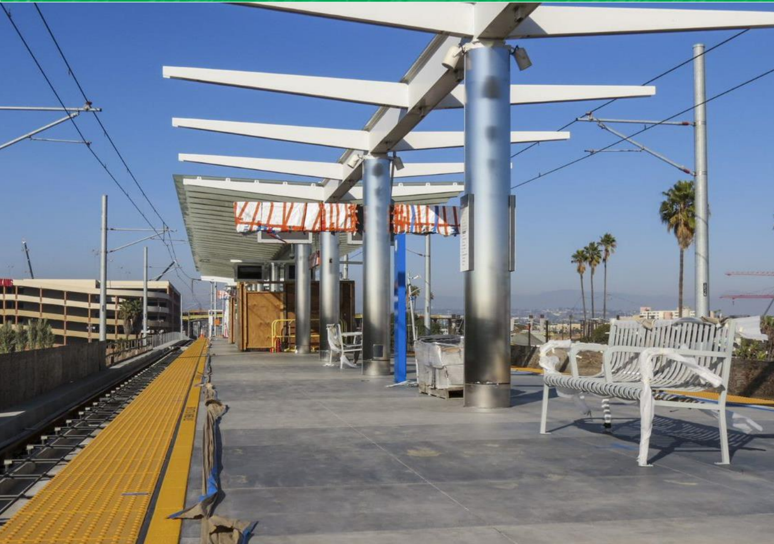
Directional signage, LED and LCD message boards, encased platform base, PA systems, and pedestrian benches
