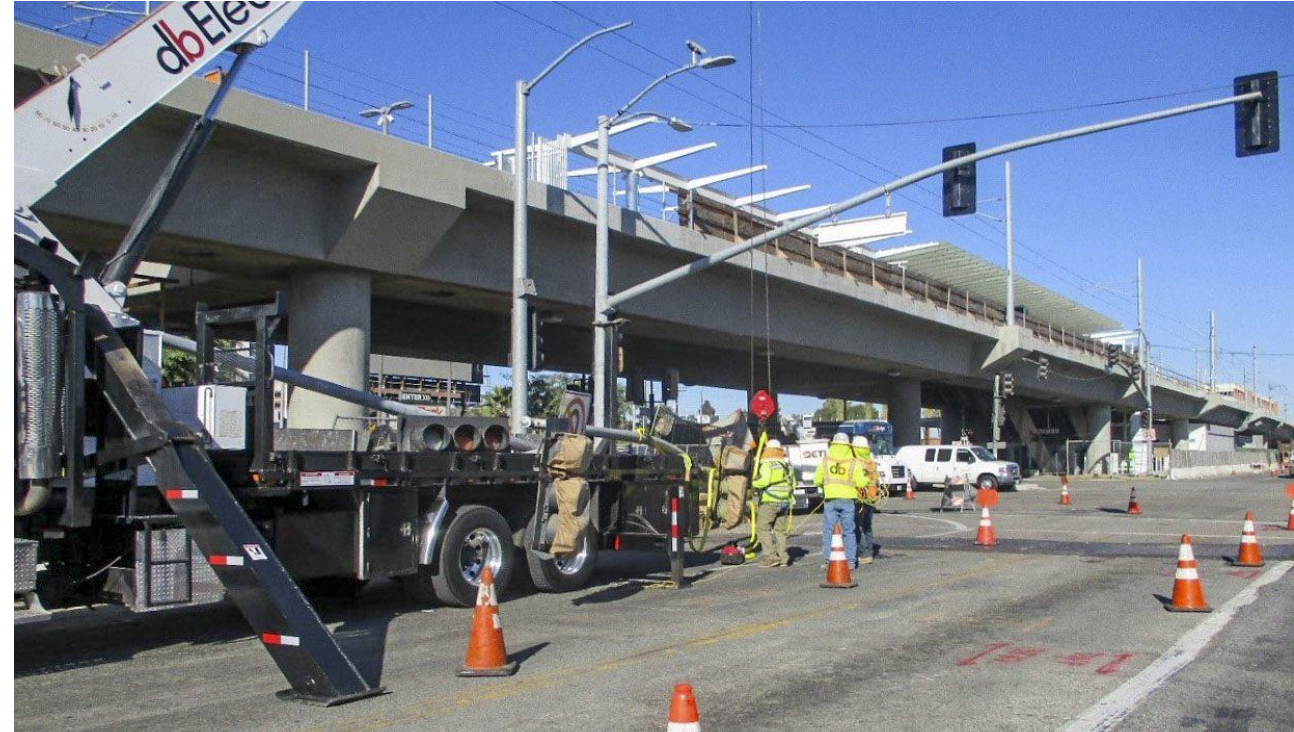
Installation of traffic lights at Aviation Bl and Century Bl
